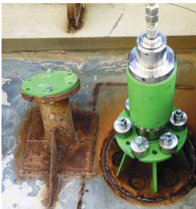
Figure 1. The Silo-Flow™ device installed on a feeder bin (next to a pipe of a dismantled air cannon).
